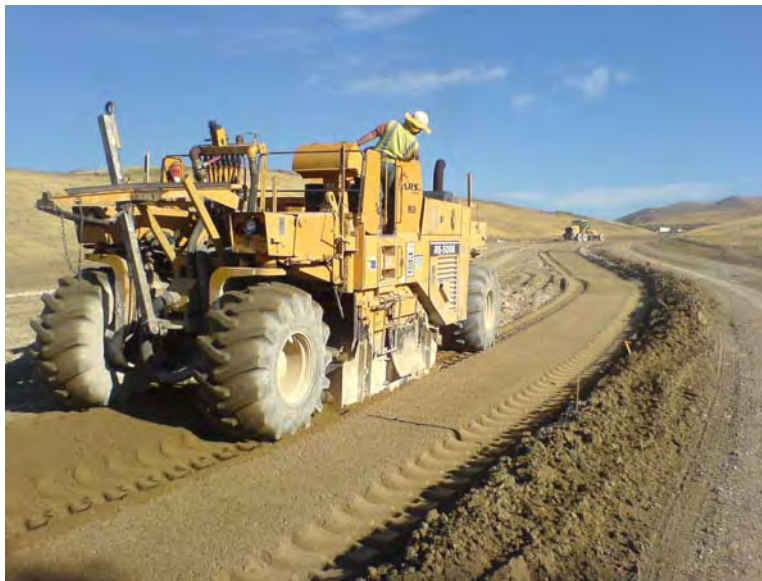
Figure 3-1. Final field mixing of lime-treated soil 1
